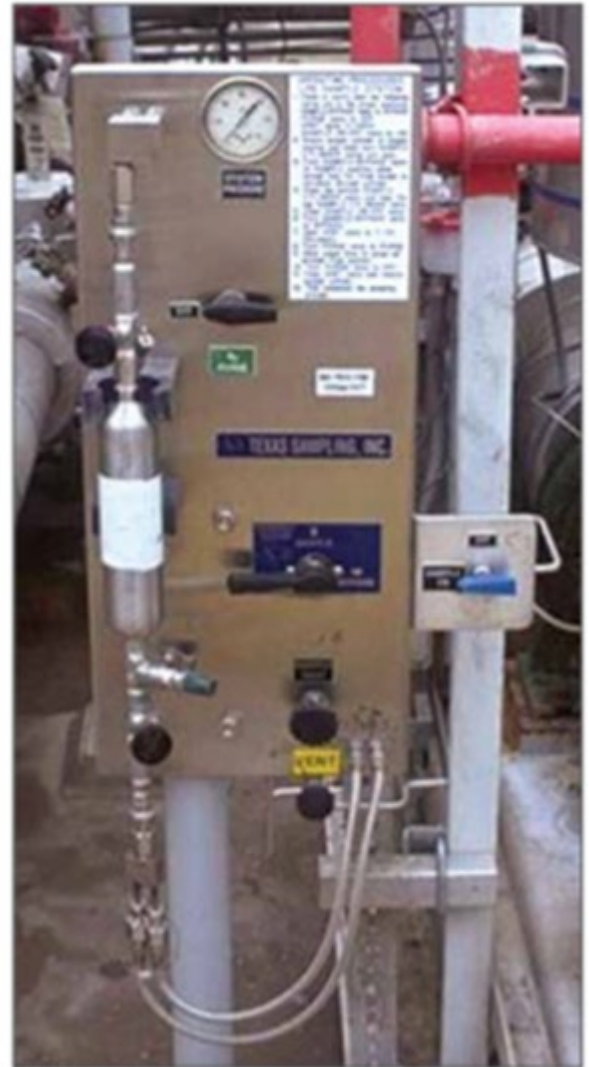
Typical sample panel system used for ethylene oxide sampling. (Ethylene Oxide Panel/ Ethylene Oxide Safety Task Group, 2007, p.67)
